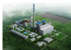
3x600MW Sumsel 9&10 Power Plant
