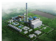
2x110MW Banjarsari Power Plant
