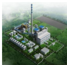
2x620MW Banko Tengah (Sumsel 8) Power Plant
