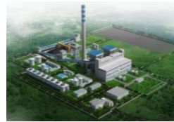
2x350 MW Kuala Tanjung Power Plant
