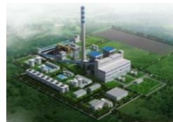
2x300 MW Sumsel 6 Power Plant
