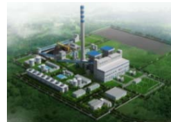
2x620 MW Banko Tengah (Sumsel 8) Power Plant
