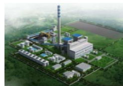
2x40 MW Halmahera Timur Power Plant
