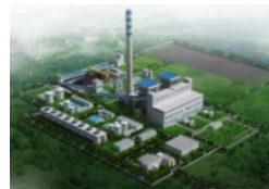
2x300 MW Peranap Power Plant
