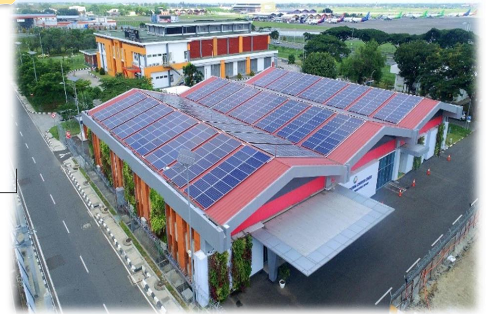
In AOCC (AirPort Control Operation Center) building Soekarno Hatta Airport COD October 2020
